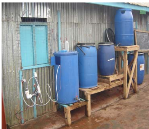
Water filtration unit built during this year's mission trip.
